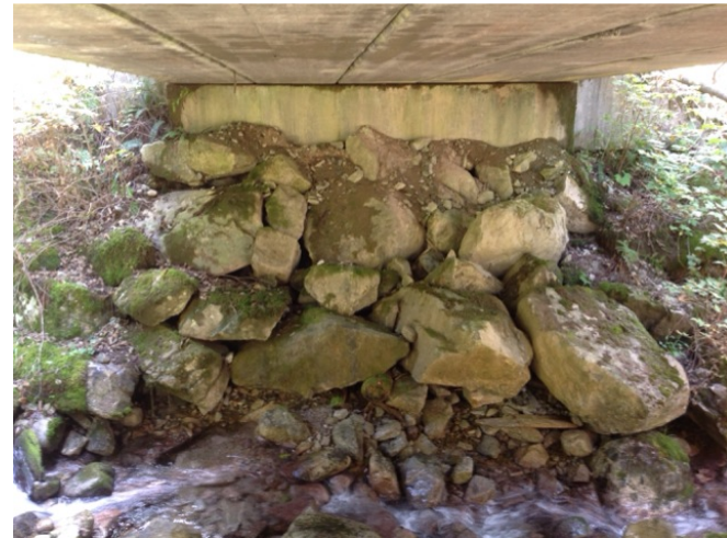
Left Bank Abutment when facing downstream
