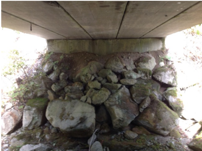
Right Bank Abutment when facing downstream
